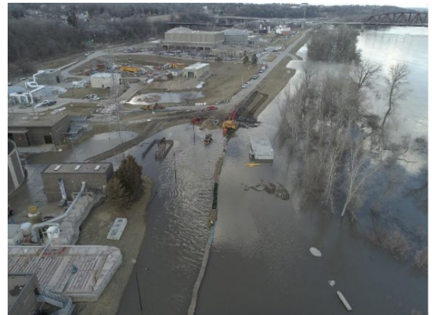
Missouri River Water Resource Recovery Facility, Omaha, NE (Temporary Levee – 2021)
